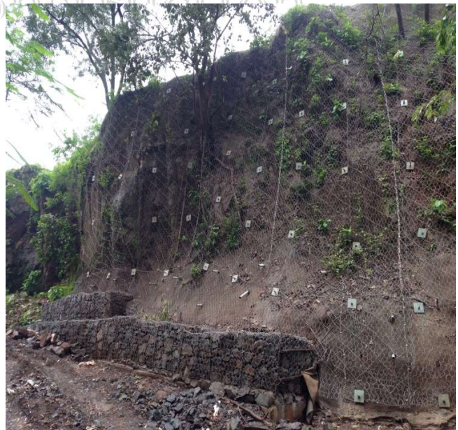
Fig:01 Anchored rock & Gabion
