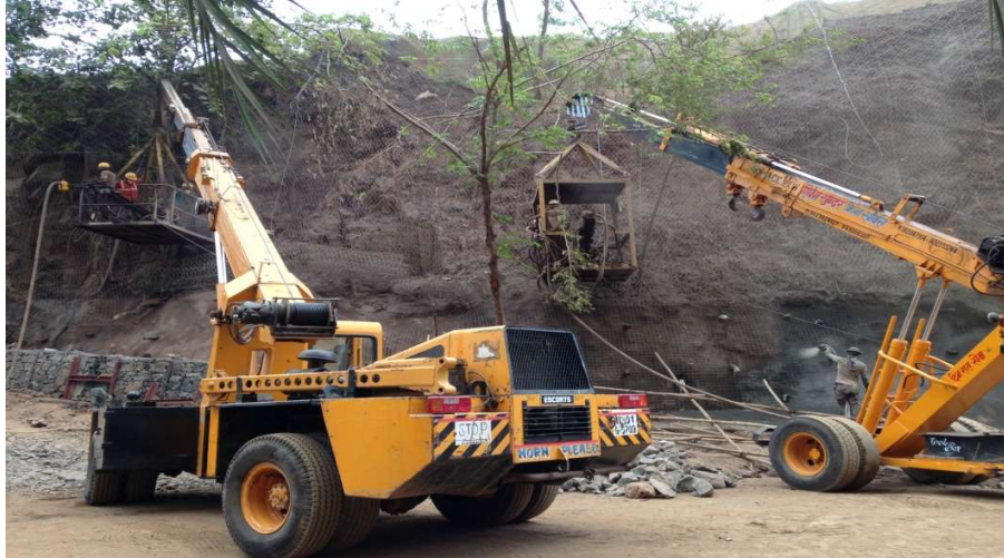
Fig:06 Multitasking SHOTCRETE-GABION-DRILLING
