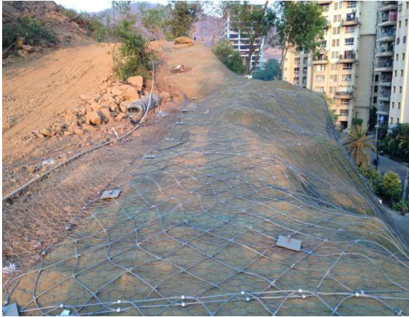
Fig:02 Coir Mat on slopes
