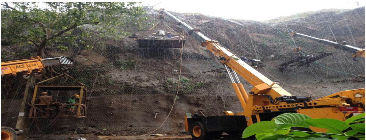
Fig:05 Drilling at Various Heights
