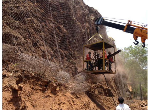
Fig:03 Drilling to 15mts Depth
