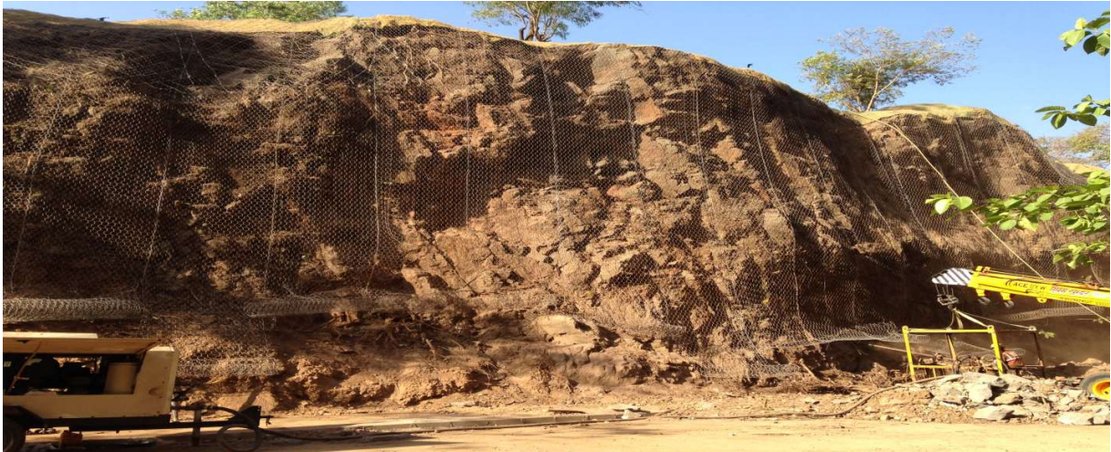
Fig:04 Laying of DT Mesh
