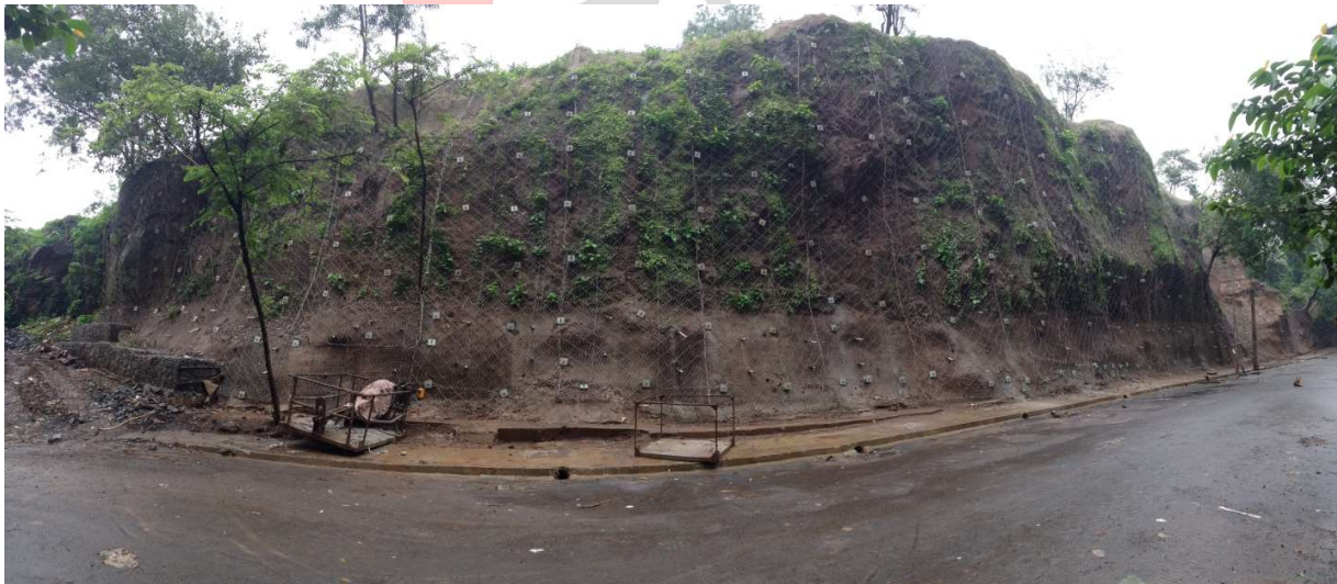
Fig:06 Completed Rock Anchoring and Rockfall Protection Structure
